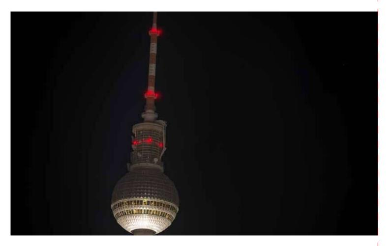
Obstruction lighting is crucial to tall structures, buildings, and airports around the world. A legal requirement, it marks the presence of all tall structures that may be a hazard to air navigation at night. The lighting system must be designed to meet International Civil Aviation Organization (ICAO) standards for product specification and placement to meet the highest levels of safety and visibility.
